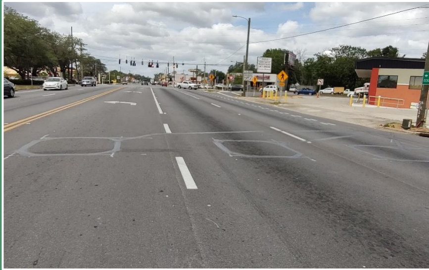
Type B inductive loops provided for advanced detection in the left turn and through movement lanes. (Marion County)
