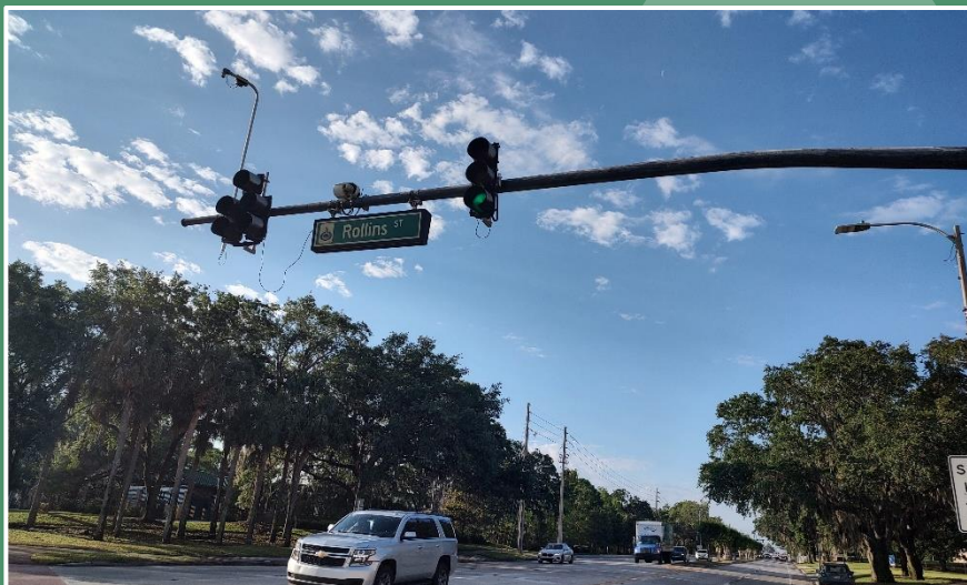
Hybrid video-radar sensors provide the ability to capture both stop bar and advanced detection zones for a single approach simultaneously. (City of Orlando)
