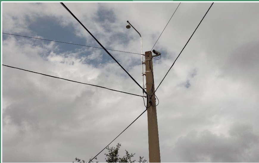
Candy cane vertical mounting arm for omnidirectional camera affixed directly to concrete strain pole for a span wire intersection. (City of Orlando)
