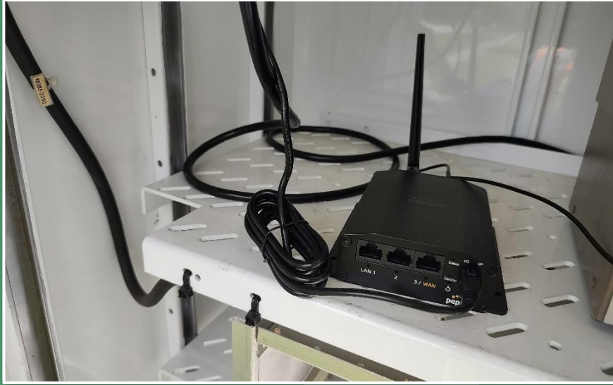
Shelf-mounted cellular modem acting as router to provide network connection between the controller and local maintaining agency network. (Lake County)
