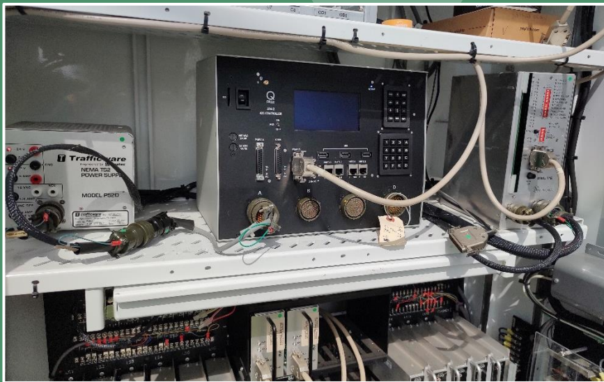
Q-Free (formerly Intelight) XN-2 ATC unit, TS-2, Type 2 model, operated as Type 1 ("A" connector only). (Lake County)
