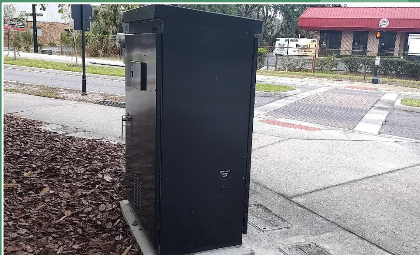
NEMA Type 6 controller cabinet assembly with matte black powder-coat finish and additional rear door. (Seminole County)
