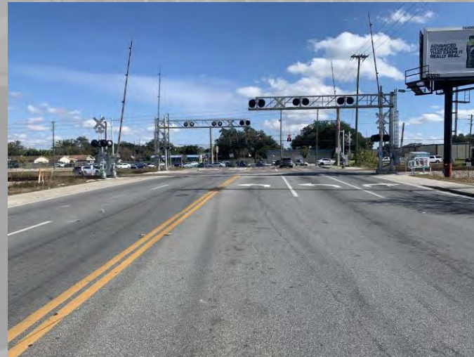
E. Lancaster Road (E.B.)
