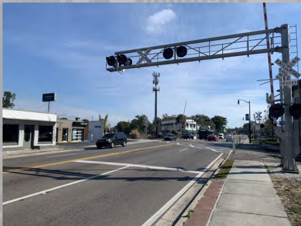
SR-426/527 / Fairbanks Ave. (E.B.)
