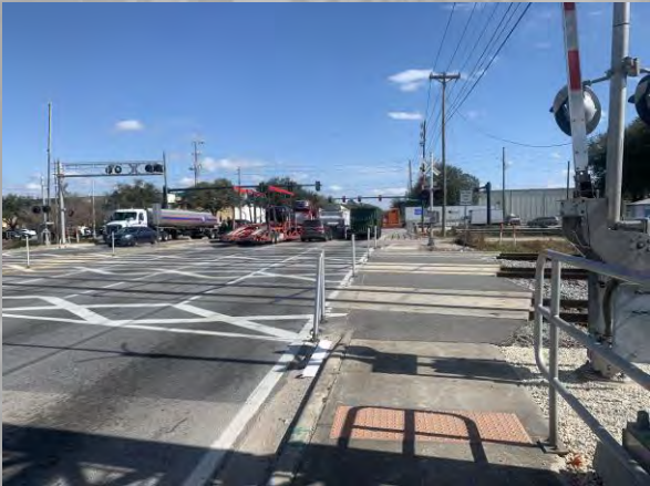
CR-528 / E. Landstreet Road (E.B.)
